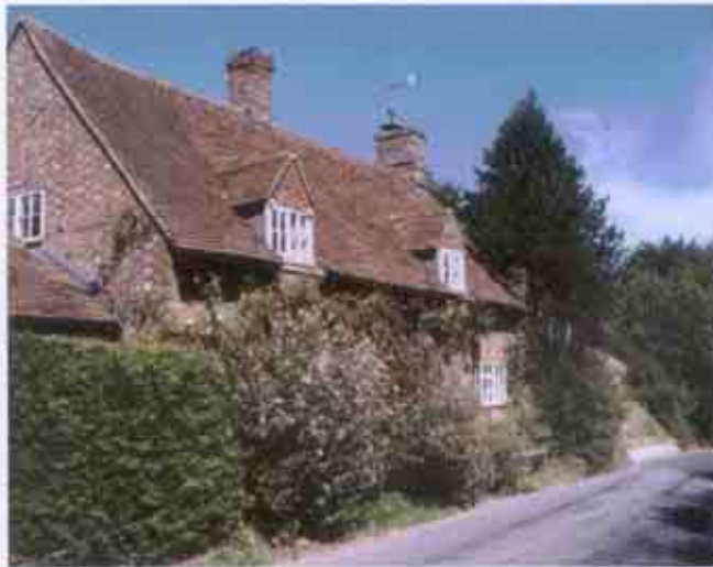
Well balanced roof pitch, positioning of dormers, and traditional brick and clay tile construction
