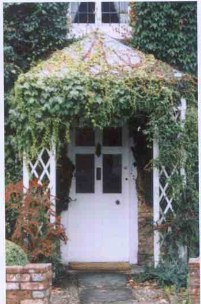
This simple porch is attractive and effective
