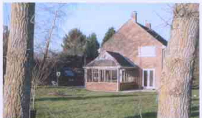
An example of a conservatory designed to fit in with the house
