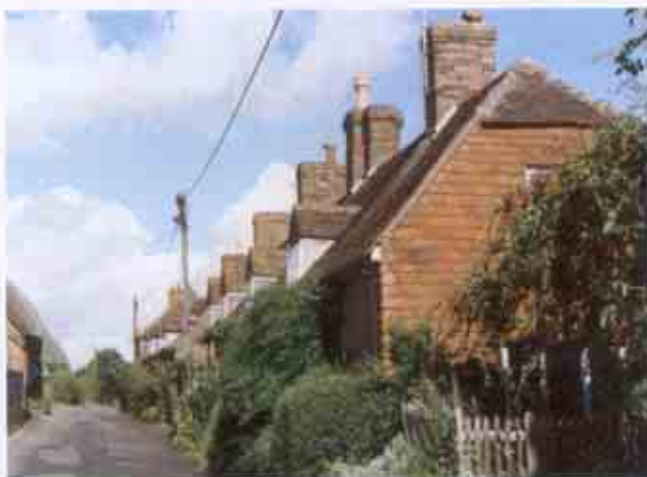
Traditional brick and clay tile construction in Farm Lane. The thatched cottages opposite date from the time of the Great Plague.
